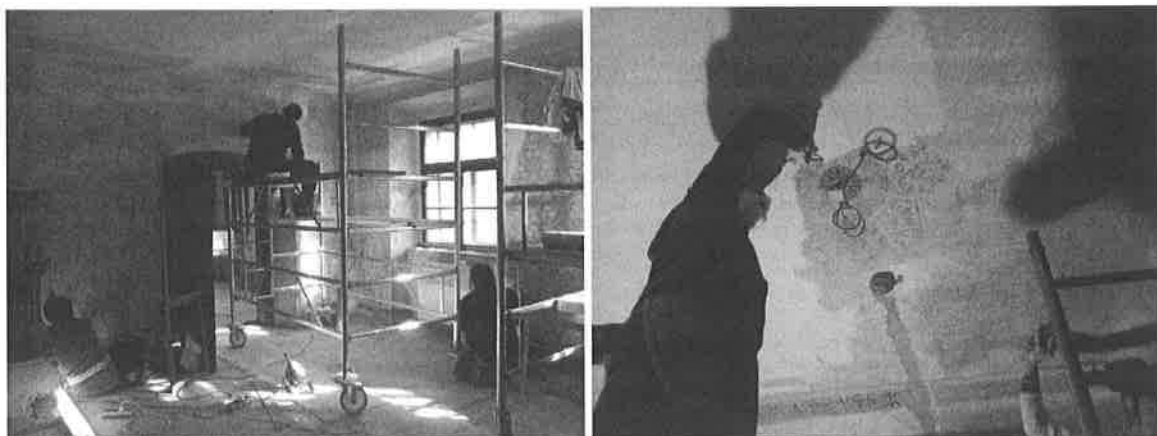
Restavratorska dela v 2. nadstropju
